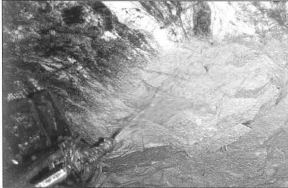
Fig. 7: TekFlex spraying at Fraser Mine
