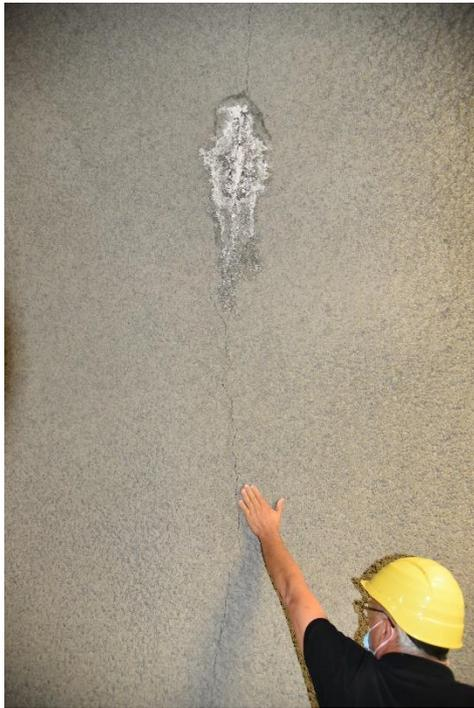
Figure 4: Crack and wet spot in Cavern 1
