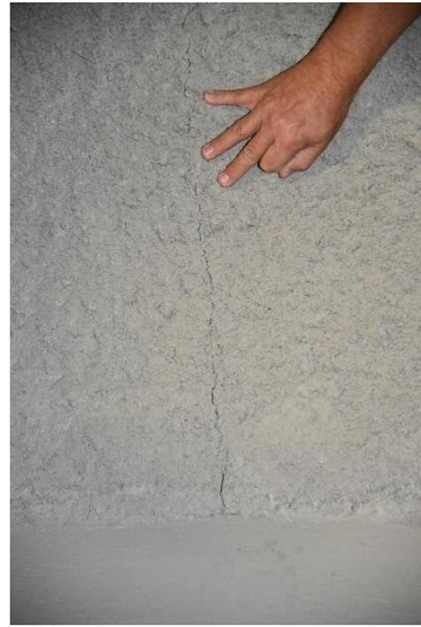
Figure 5: Crack from invert upwards (here Cavern 3) [Master Builders Solutions]
