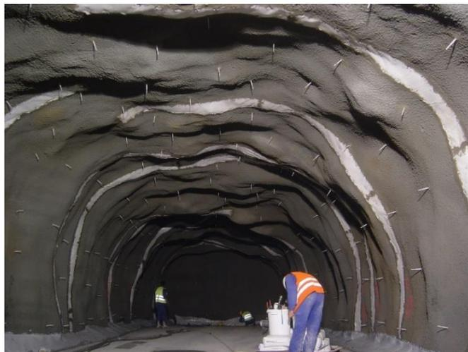
Figure 2: Substrate prepared to receive the sprayed membrane. Dripping water channeled via stripes into invert. Depth guidance pins installed for the thickness control of permanent sprayed concrete [Master Builders Solutions]
