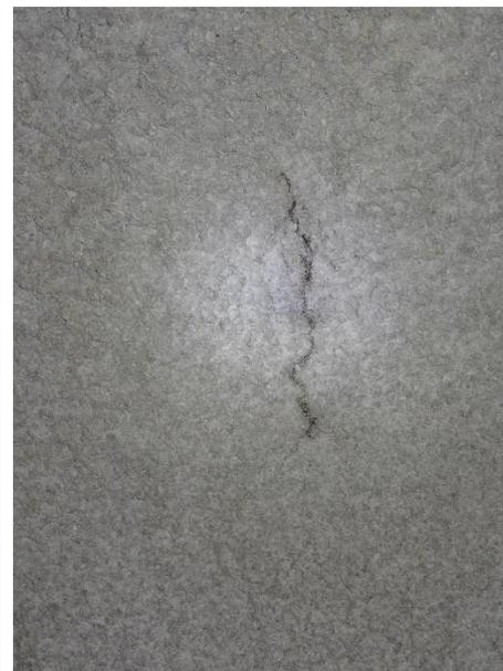
Figure 9: Small, short vertical crack [Master Builders Solutions]
