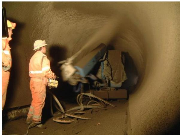
Figure 6: Wet-mix sprayed concrete application [Master Builders Solutions]
