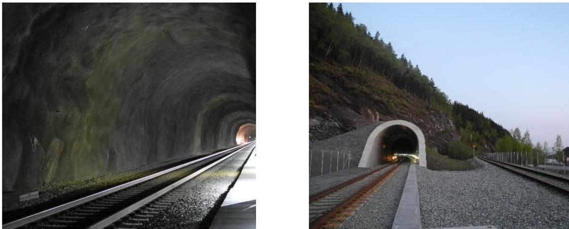
Figure 13: Gevingås rail tunnel. Left: interior of the tunnel showing a portion of the tunnel with a final inner lining of sprayed concrete and a spray-applied waterproofing membrane. Right: the northern portal with a cast-in-situ lining and showing the old rail line to the right [8]
