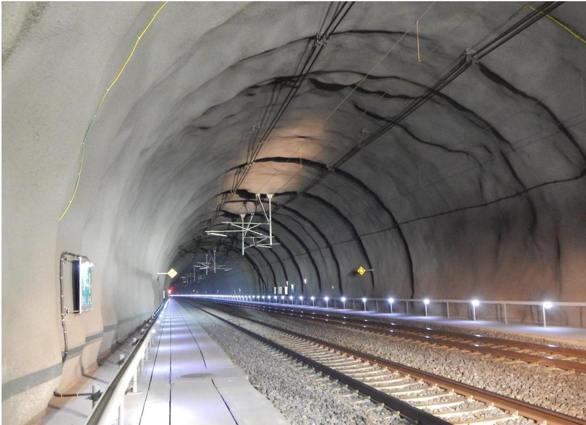
*Figure 3: In-service condition of a section of the Holmestrand railroad tunnel in Norway after three years of operation after the completed construction (2016). The lining system is permanent sprayed concrete waterproofed with a spray applied membrane in a continuously bonded structure (photo: Karl Gunnar Holter).*
